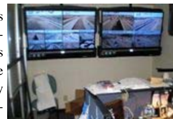
Traffic Management Center at TxDOT Amarillo District Office
