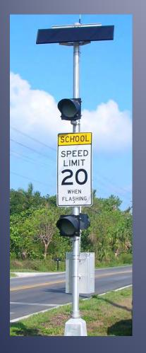
A flashing beacon indication for speed reduction notification during specific periods of school operation.
