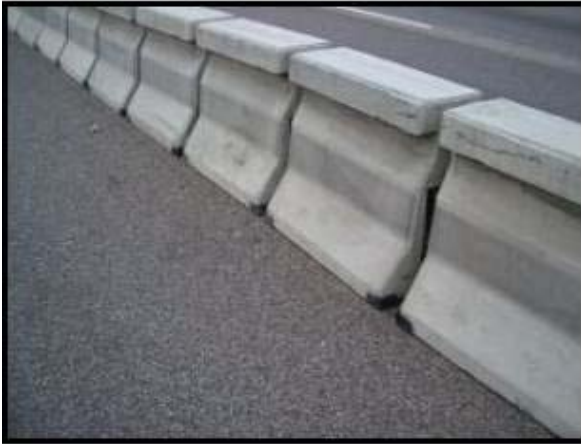
Concrete Barrier Sections Barrier Transfer Machine
