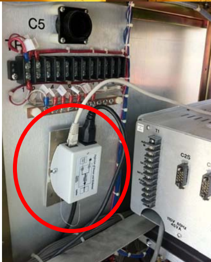
POE unit mounted in traffic cabinet
