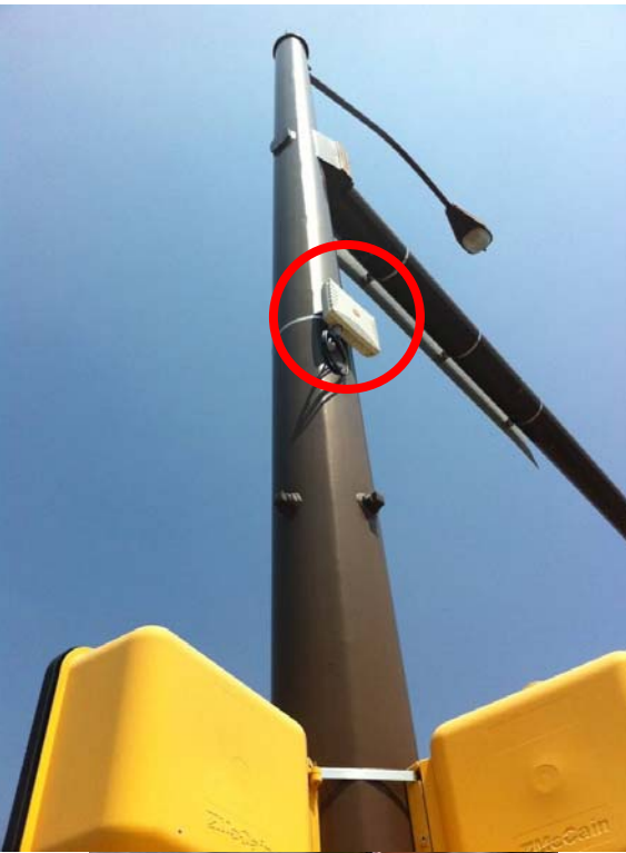
Modem mounted 15 ft high on pole closest to our cabinet
