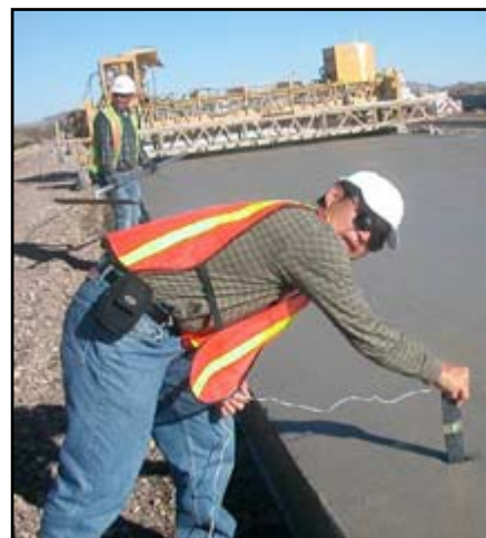
Placement of Flexi-Probe in still-wet concrete.
