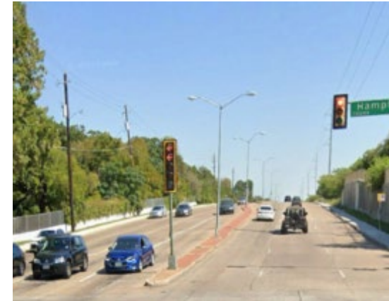
Absence of striped crosswalks at S. Hampton Road
