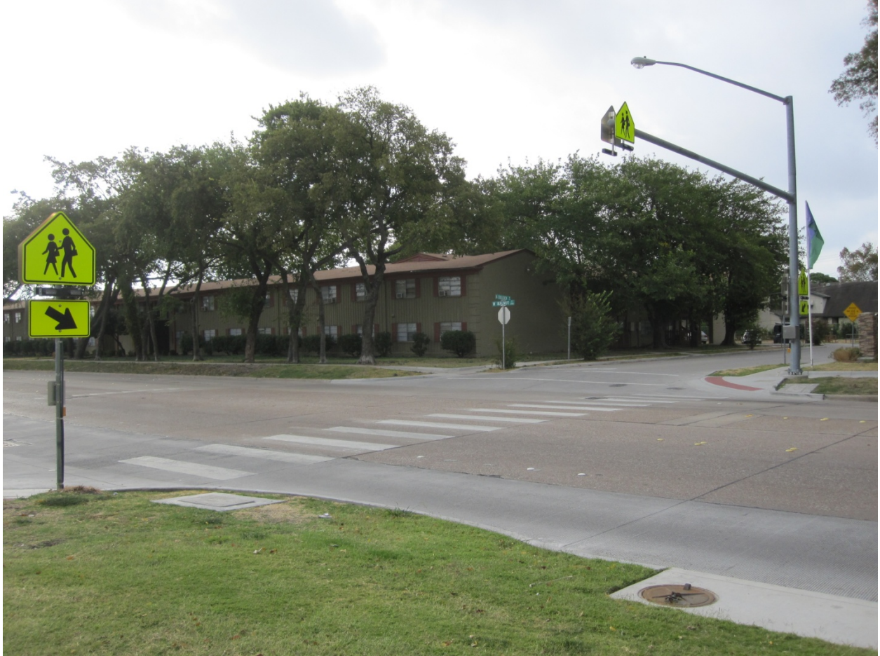
Figure 3. Crosswalk After Installation of RRFB.
