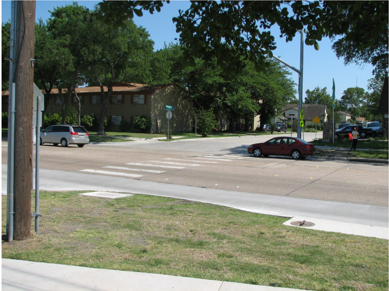
Figure 2. Crosswalk Prior to Installation of RRFB.
