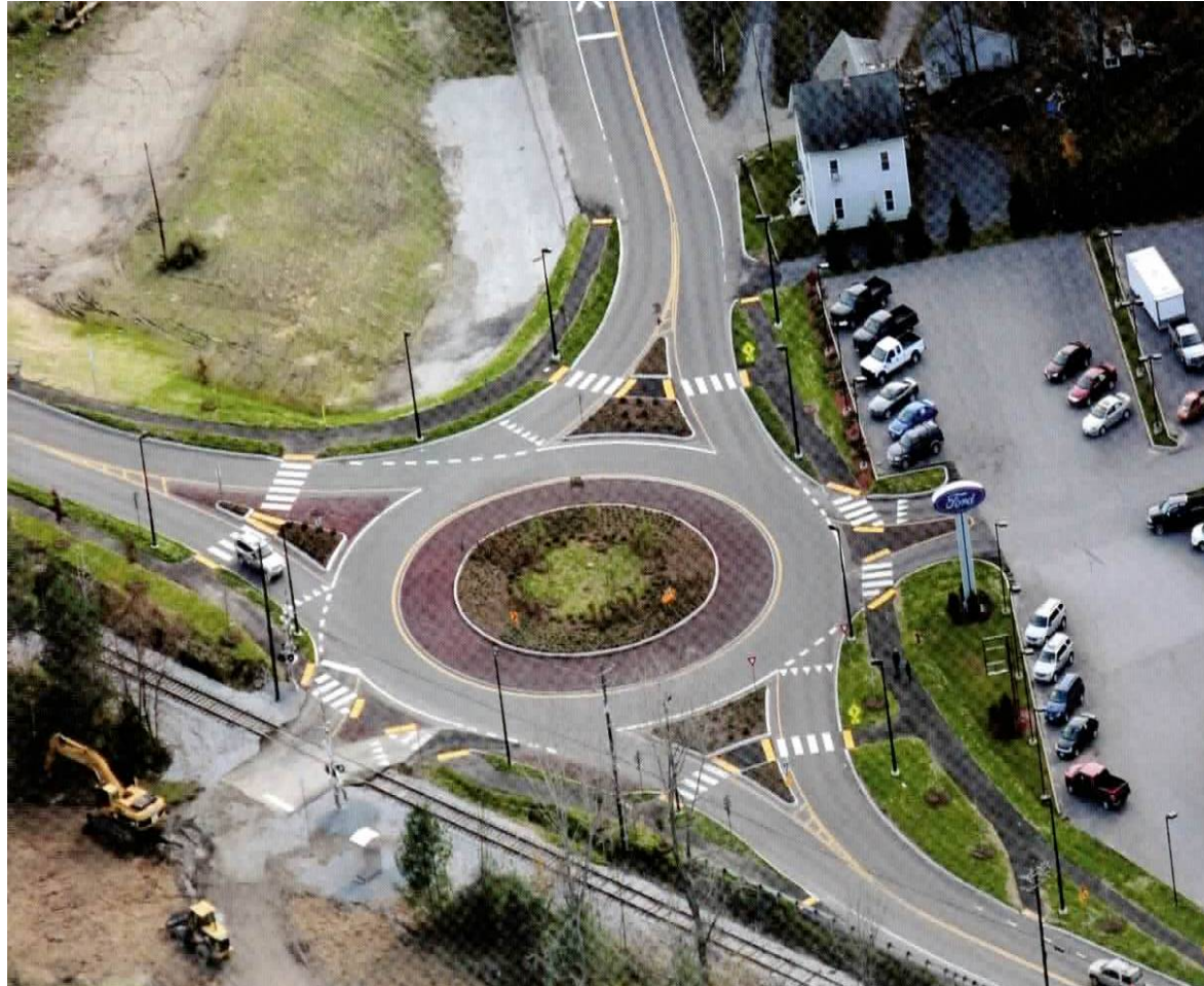
US 2 & US 302 Roundabout – Montpelier, Vermont (Image courtesy of City of Montpelier, Vermont)
