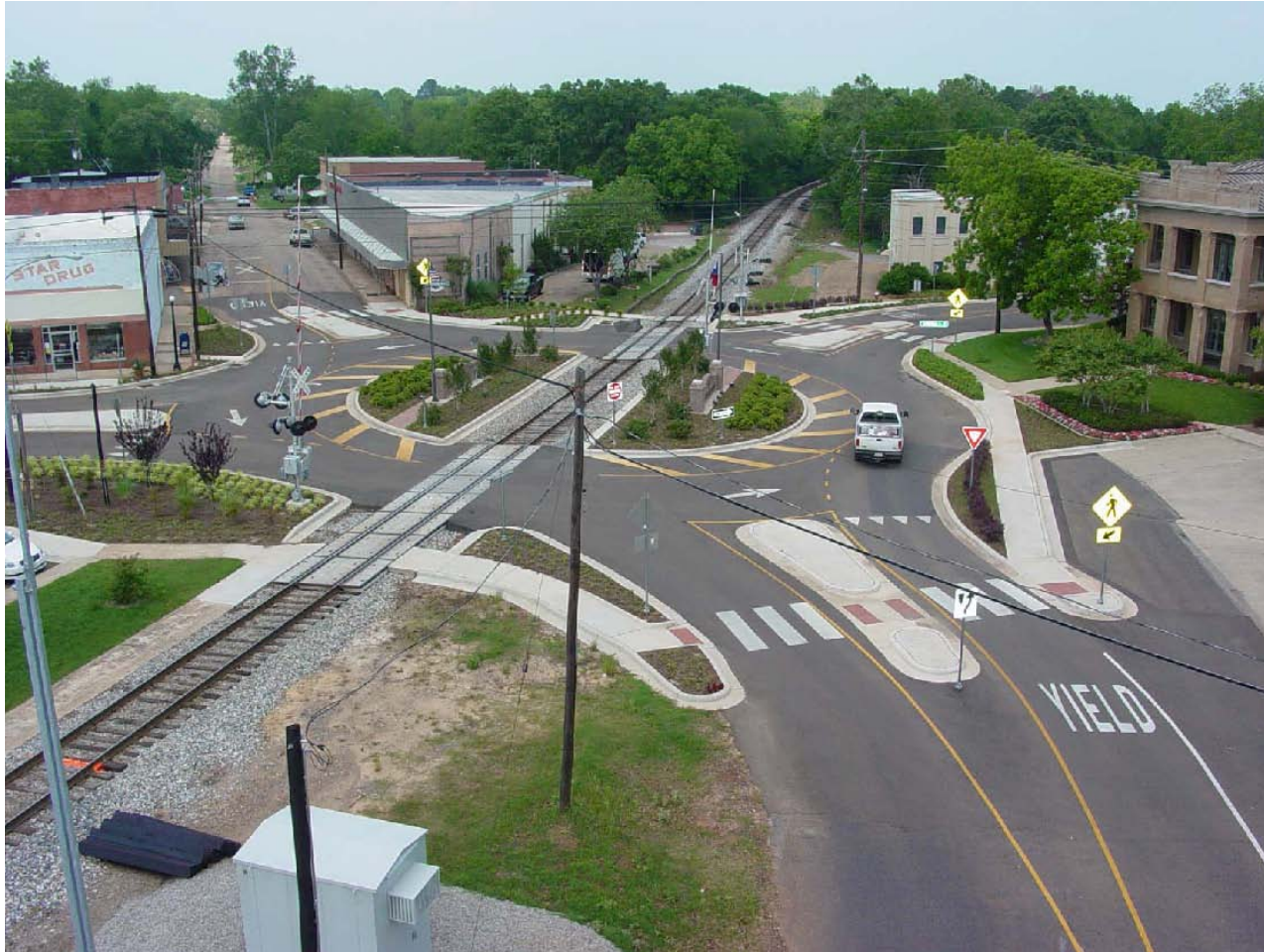
Jefferson/Webb/Coffey Roundabout – Daingerfield, Texas (After) (Image courtesy of Brown & Gay, Inc.)
