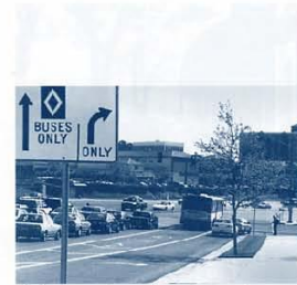
This bus by-pass lane and signal priority in San Diego allows transit to move easily through a congested intersection.
