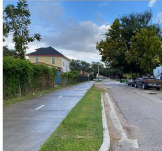
CG-1.2 Built example of multi-use pathway one side of the street in Houston
