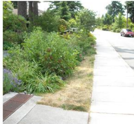
OD-3.1 Built example of permeable sidewalk on one side of a one-way street
