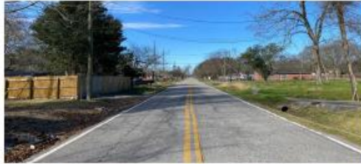
Typical existing conditions on local residential streets
