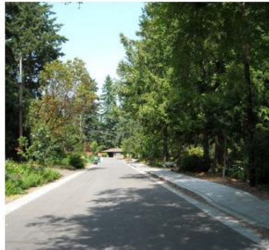
OD-2.3 Built example of reggraded street with concrete sidewalk and a consolidated bioswale on one side of the street
