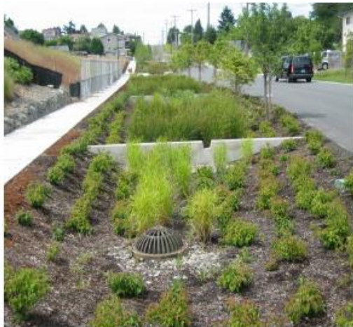
OD-1.0 Built example in Seattle, WA Photo courtesy of Mark Holema
