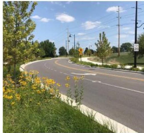
OD-1.0 Built example in Eagle Creek Photo courtesy of Ecologic
