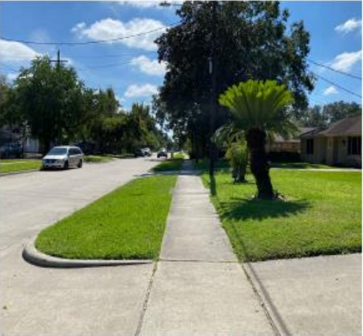
CG-1.1 Built example of landscape buffered standard concrete sidewalk in Houston
