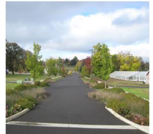
OD-1.2 Built example of porous asphalt in Pringle Creek; Photo courtesy Greenworks
