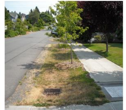
OD-1.1 Built example of permeable sidewalk in Seattle, WA
