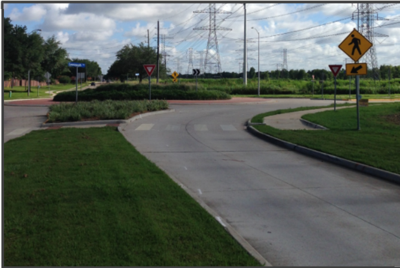
Commonwealth Blvd and LJ Pkwy roundabout, Sugar Land TX
