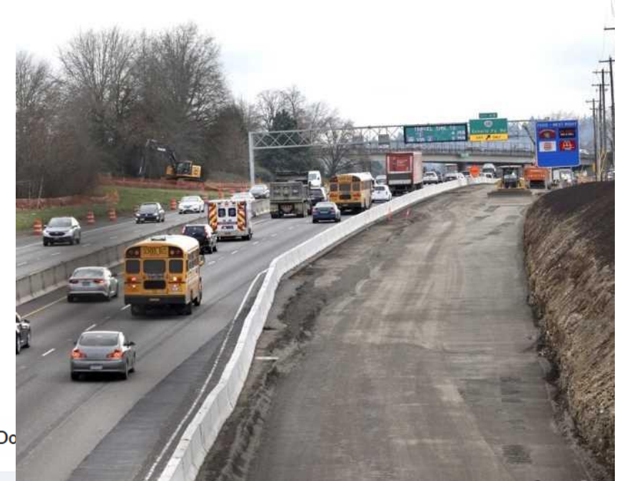
Source = Portland Tribune, https://pamplinmedia.com/sg/77-news/537674-430630-officials-tout-highlights-of-highway-217-improvements
